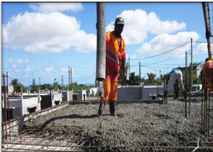
Roof Slab Grant
