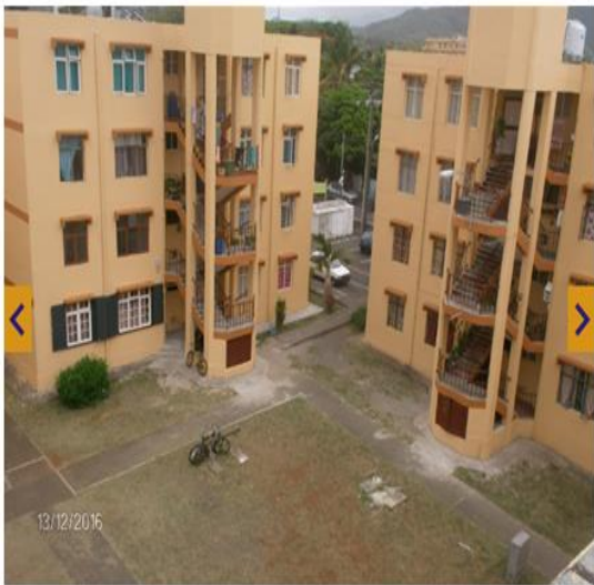
Beau Vallon Housing Estate after rehabilitation
