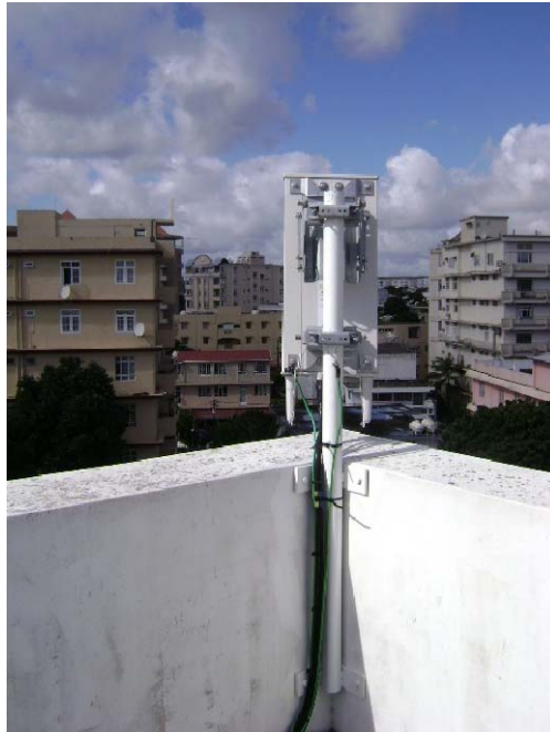
Figure 5: Example of a De Minimis structure
