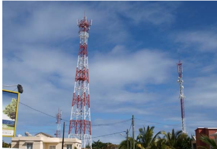
Figure 1: Standalone lattice steel structure
