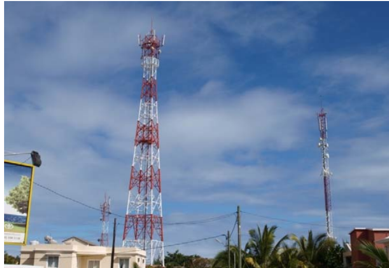
Figure 1: Standalone lattice steel structure
