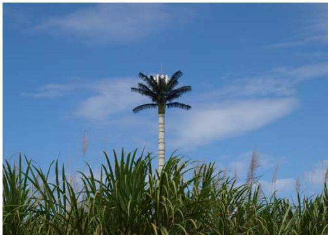
Figure 4: Stealth design techniques
