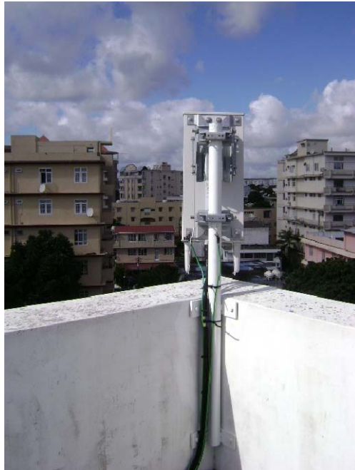
Figure 5: Example of a De Minimis structure
