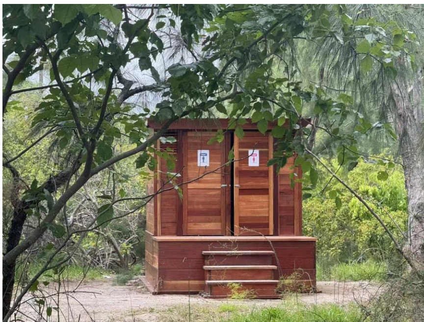
Figure 19. Improper use of the dry toilets causing hygienic and sanitation issues, including foul smell and flies' nuisances
